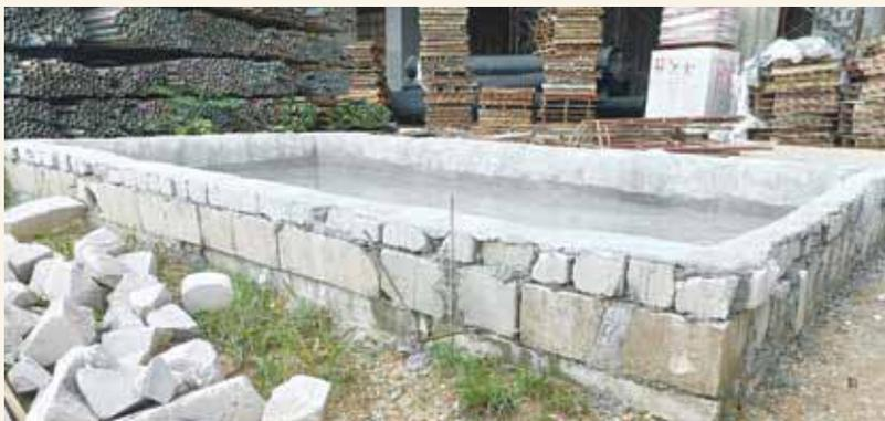
Surplus bricks are reused as bunds to prevent oil spillage from the IBC tank
