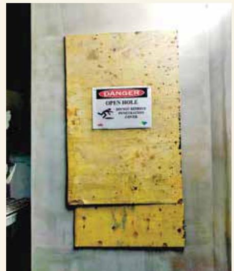
Used plywood is repurposed and used as coverings for penetration or void holes.
