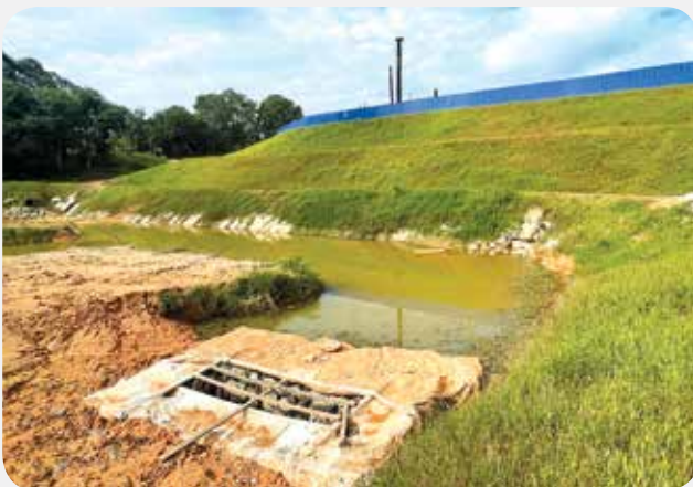
Silt traps at W City Larkinton
