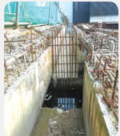
Rubbish and debris traps at the perimeter drainage at 118 Mall project site
